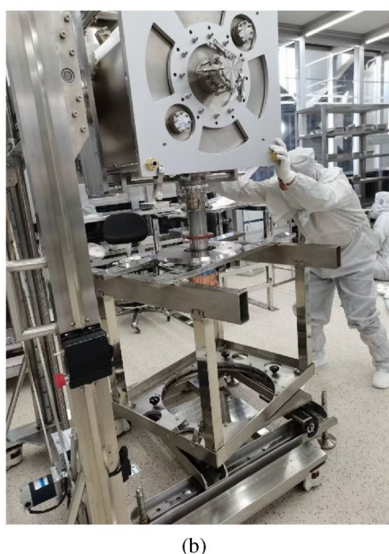
Fig. 18 (Color online) Installation of the jacketed cavity and the coupler. (a) 3D modeling; (b) actual installation
