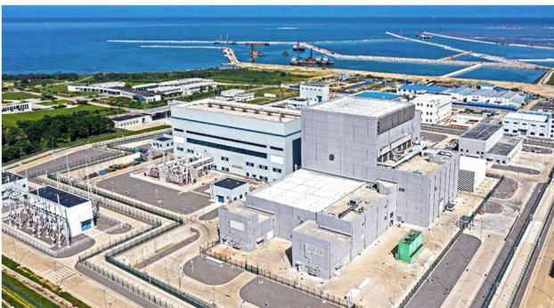
**Fig. 1** (Color online) 200 MWe HTR-PM high-temperature gas-cooled reactor nuclear power demonstration plant in Shidao Bay, Shandong Province, China
